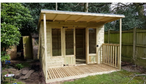
STEP 5: Shed Construction
